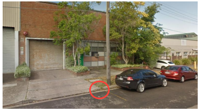
Figure 5: Kerb Outlet 3 (source: Google street view)
