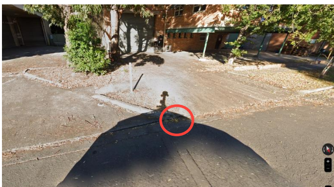
Figure 10: Kerb Outlet 8 (source: Google street view)
