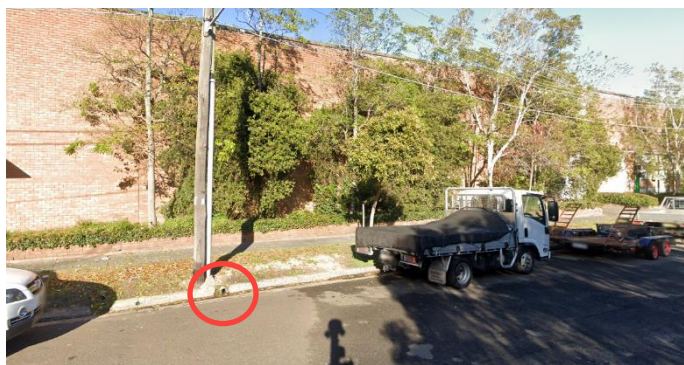
Figure 8: Kerb Outlet 6 (source: Google street view)
