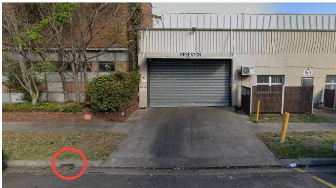
Figure 4: Kerb Outlets 1 & 2 (source: Google street view)
