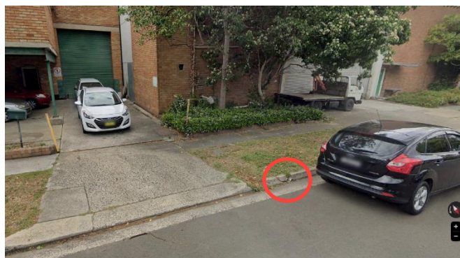
Figure 9: Kerb Outlet 7 (source: Google street view)
